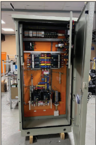
AUTO TRANSFER SWITCH PANEL (ATS)
