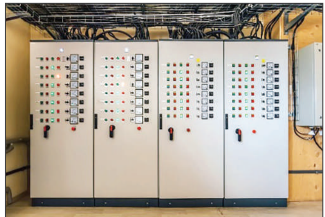
MOTOR CONTROL PANEL (MCP)
